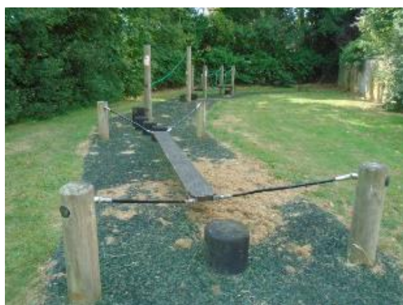
Trailblazer – splits/cracking in timber, listed a “limited life unit”
