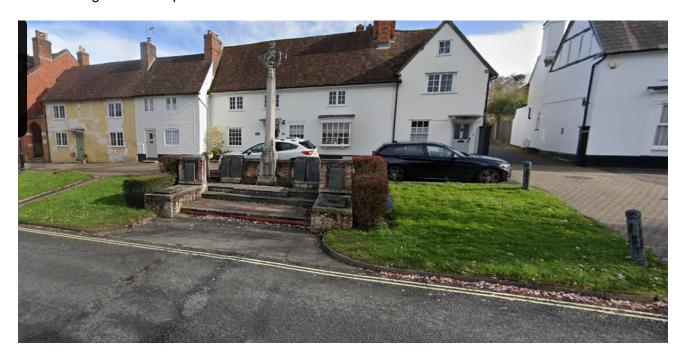
OPC carried out work in 2020 to improve the stability of the steps. The works involved repairing several steps and curb stones and re-pointing sections of the wall.
