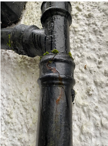
Cracked cast iron downpipe, and gutters loose in joints causing water to leak over the wall below,
