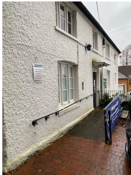
Ramp to entrance partially covering vent to timber floor being: Risk of decay. Damp dripping from leaking gutters above.
