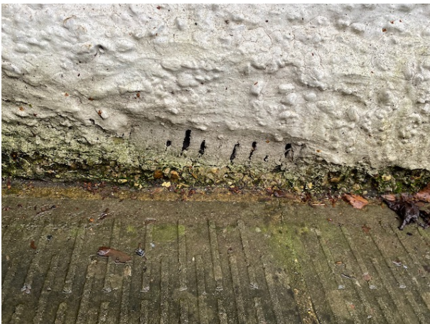
Ramp to entrance partially covering vent to timber floor being: Risk of decay. Damp dripping from leaking gutters above.
