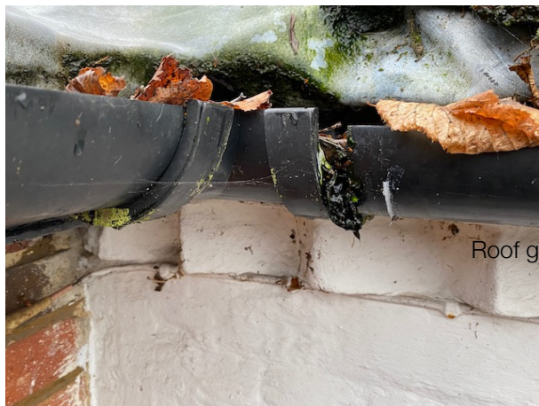
Cracked cast iron downpipe, and gutters loose in joints causing water to leak over the wall below,
