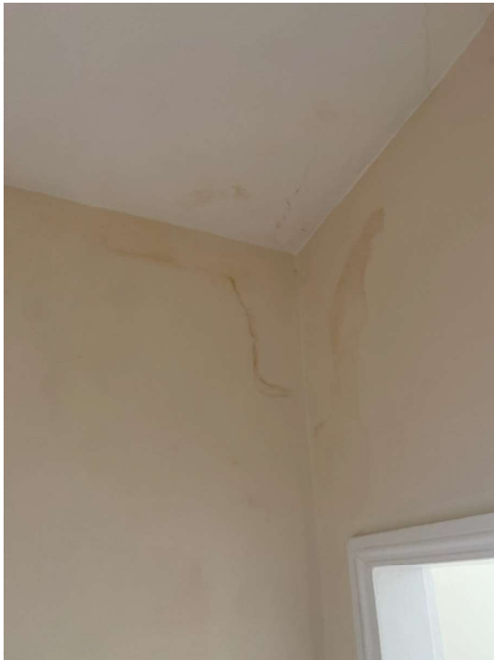
Water damage around chimney breast in main bedroom
