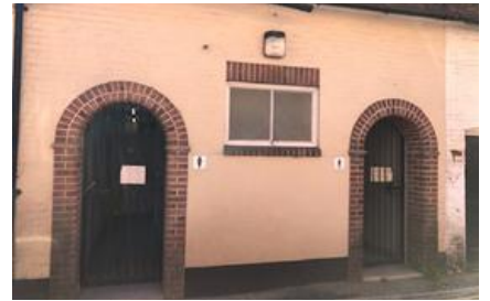
The public toilets in King Street were transferred from Hart District Council in 2012 and are now managed within Precept to provide public toilet provision, supporting High Street businesses and local events.
