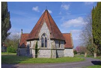
The North Chapel has undergone several repairs in recent years including installation of false wooden floor to protect the original tiled flooring from further damage. It is now used for storage of event equipment by the Council, InOdiham and the Odiham Society which is loaned for other community events.
